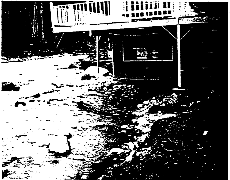
Home located on the Raging River in King County. This home is located outside the flood hazard area identified on the existing FIRM.
